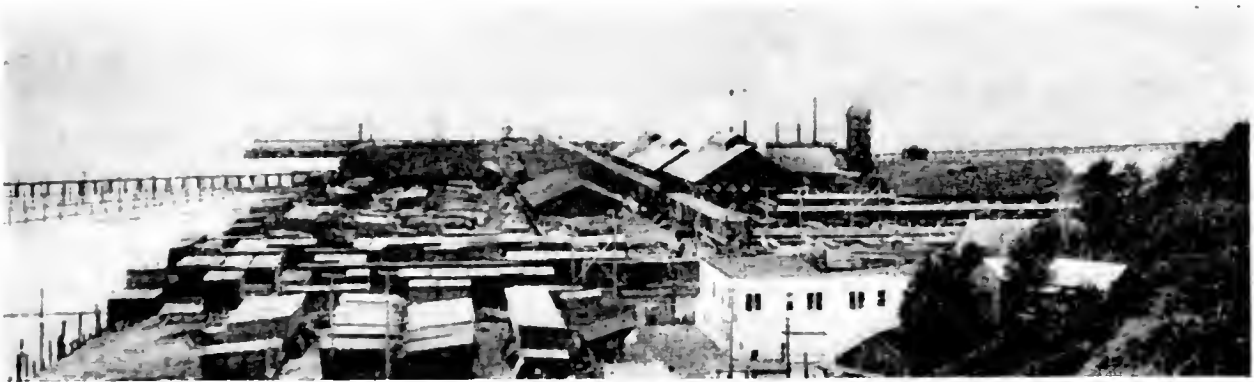
Steam Turbine Generating Plant of Hammond Lumber Company near Astoria - 1910
